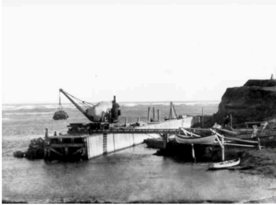
Heads wharf being constructed in May 1884. (Harding & Denton Collection, Wanganui District Library, NZC2.1.271 (Source: Dodd, 2021))
