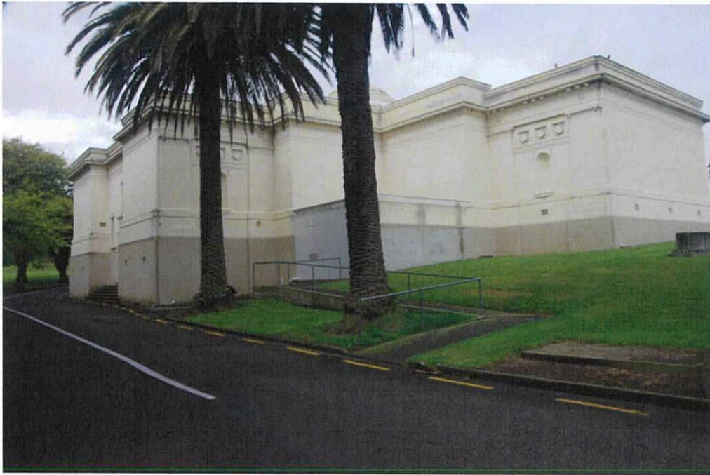
Figure 6: Looking south towards the back of the gallery. The existing loading bay (the square grey addition to the gallery), path and road will be removed and backfilled. A new footpath and bike park is planned to be built here.
