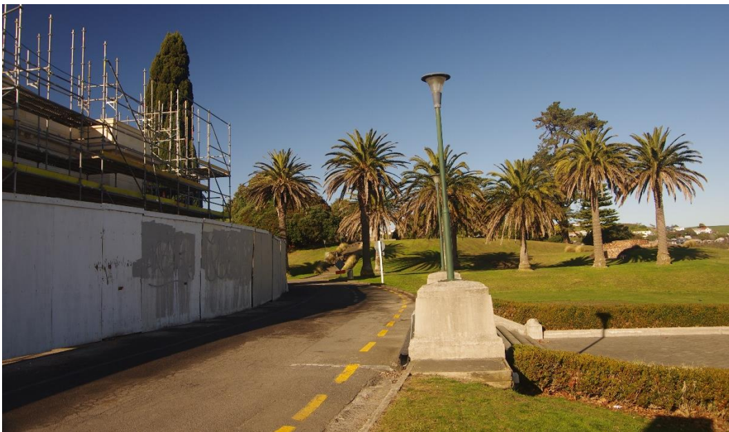
Figure 17: Showing Location Two, being the proposed location of trenching for the installation of lighting & security camera cables, in Pukenuamu Drive outside the original SAG main entrance & the top of the Veterans' Steps. The location is where the Lion Monument was built over the trench in which the remains of the soldiers were buried after they had been exhumed from their graves at Nukumarua where they were killed in fighting in 1865 (Archaeology North Ltd.).
