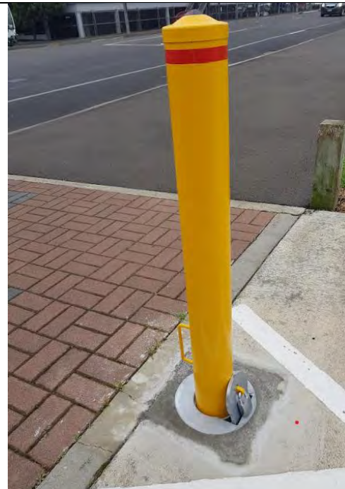
Propose all new bollards are removeable, like this one near Trafalgar Square.
