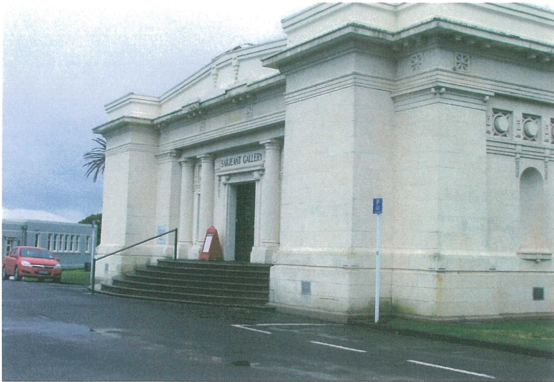
Photograph 1: The ground beside both front corners of the gallery (under grass and tarseal) will be affected by the construction of ramps and associated works.
