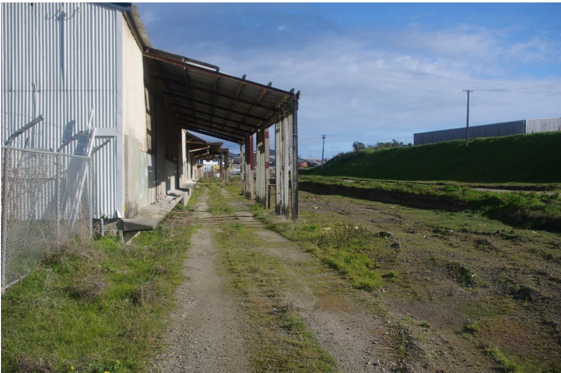
Figure 94: Victory shed with awning and siding along northern wall, looking west (15.07.2021)
