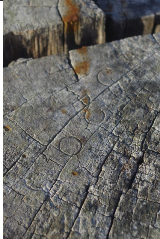
Figure 55: Detail of previous image (15.07.2021)
