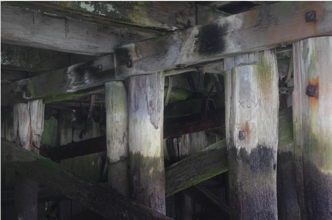
Figure 71: No.3 wharf incised roman numerals to indicate depth of driven piles (15.07.2021)
