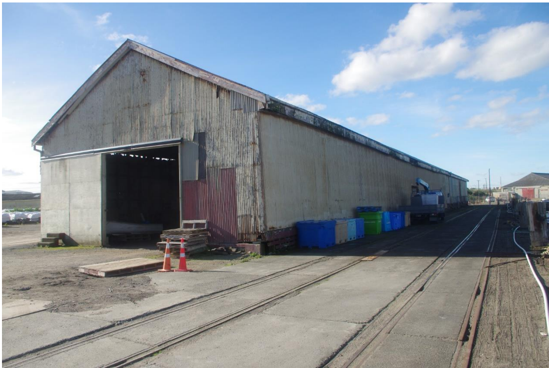
Figure 64: Red shed prior to removal, looking northeast along southern side (30.07.2020)
