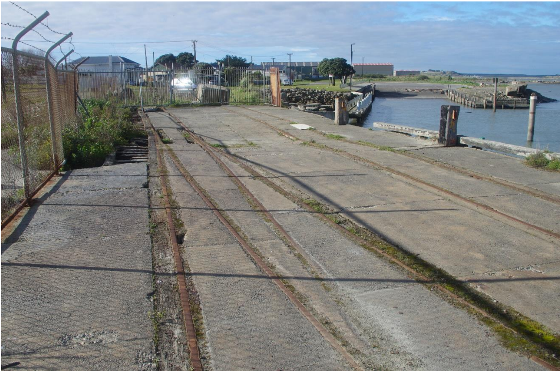
Figure 92: No.3 wharf concrete decking and embedded rails, eastern end (15.07.2021)
