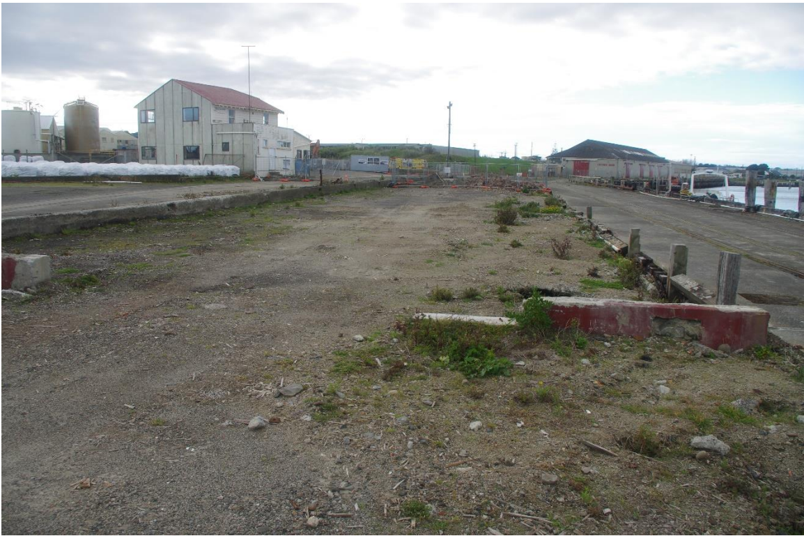
Figure 66: Red shed foundations, Victory shed in background right of frame (15.07.2021)
