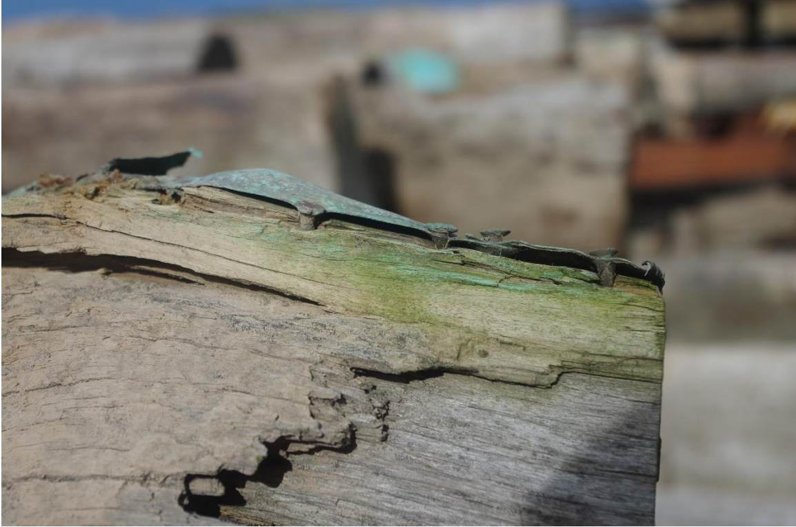
Figure 57: Details of fastenings for copper patches (15.07.2021)
