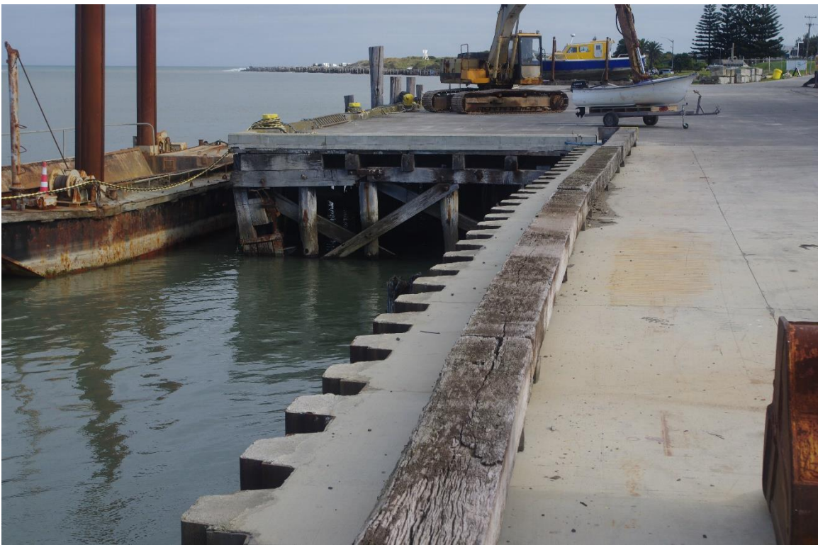
Figure 53: No.1 wharf - sheet piling repairs. Looking west towards heads (15.07.2021)
