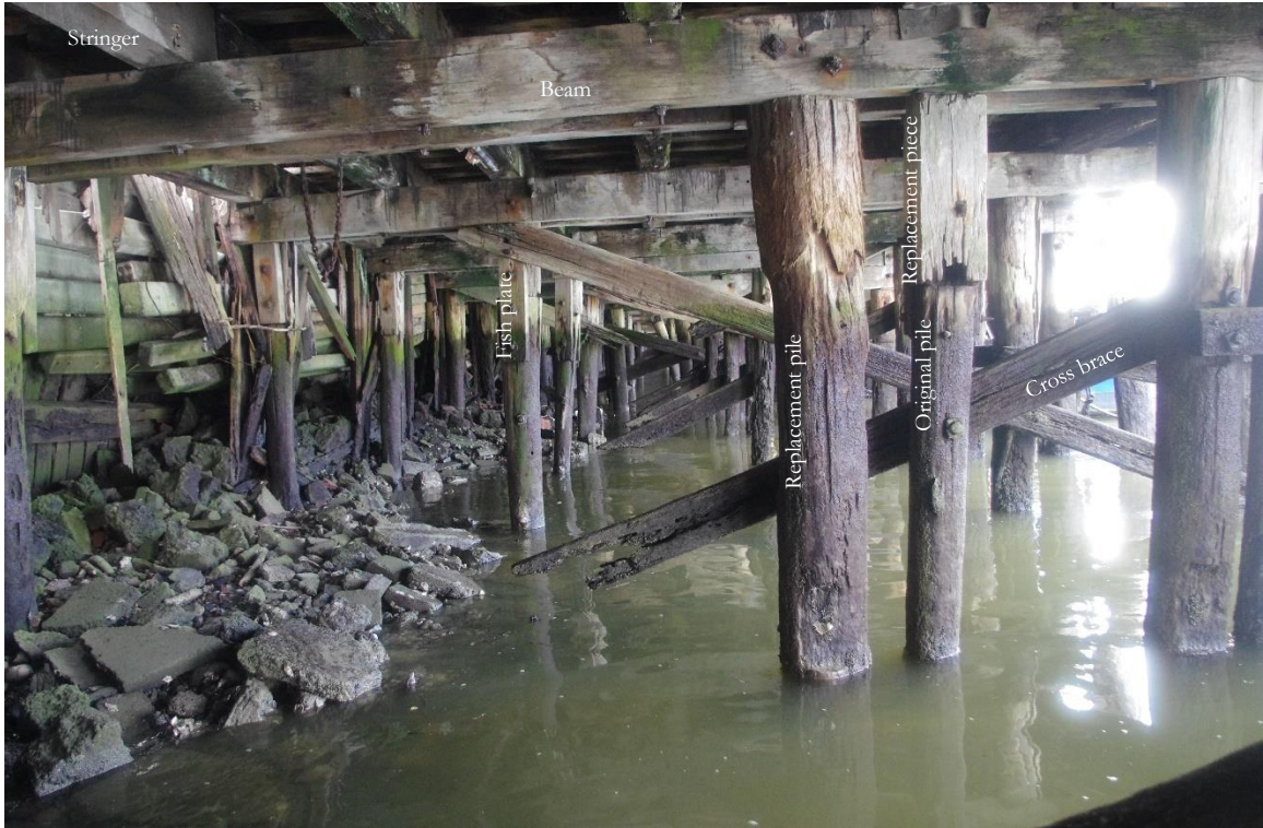
Figure 63: No.2 wharf typical arrangement of bent and repair work (15.07.2021).
