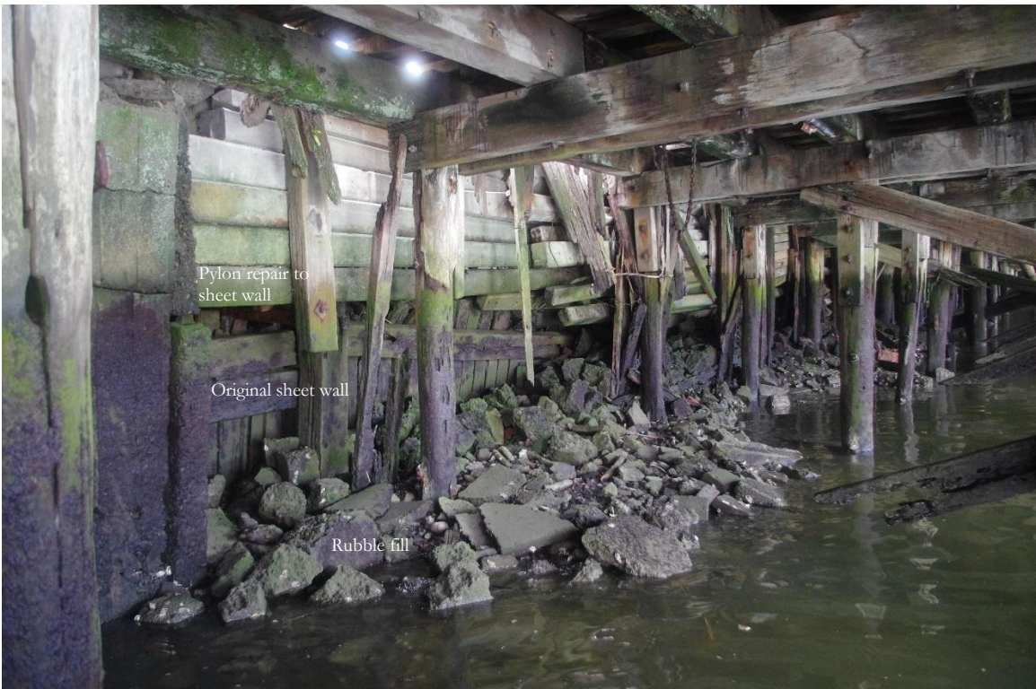
Figure 62: No.2 wharf, repairs using concrete pylons laid horizontally (15.07.2021)
