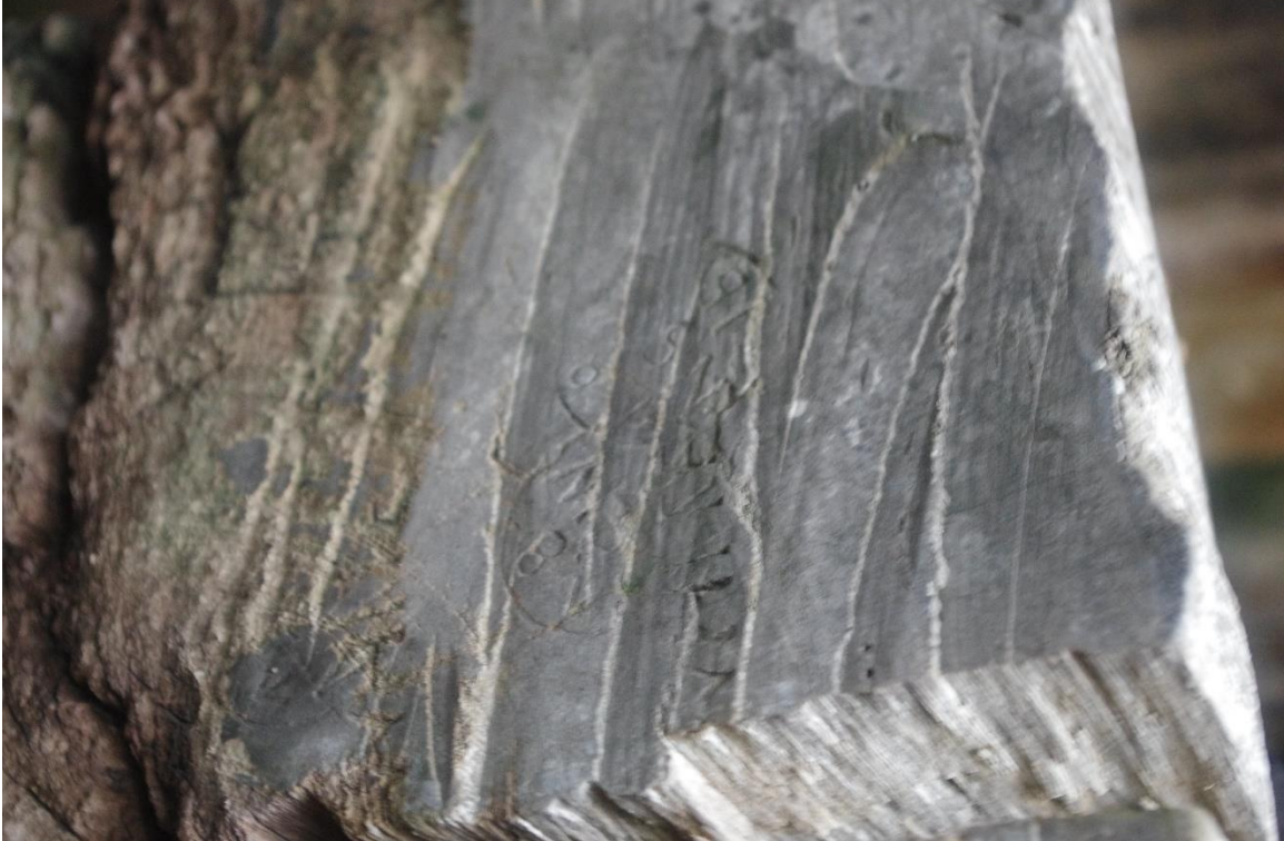
Figure 81: No.3 wharf, NSW inspectors mark (Ironbark, inspector 8) and cutters mark WHITE (15.07.2021)
