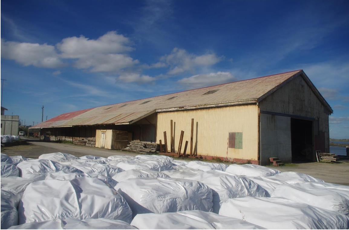
Figure 65: Red shed prior to removal, looking east along northern side (30.07.2020)
