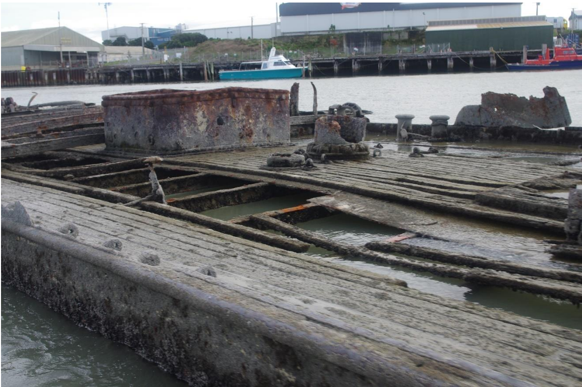
Figure 100: ss Te Anau bulk, insitu decking near bow (15.07.2021)
