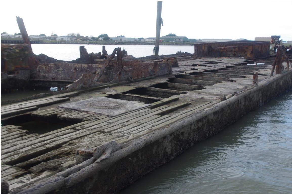
Figure 102: ss Te Anau hulk, insitu decking toward stern (15.07.2021)
