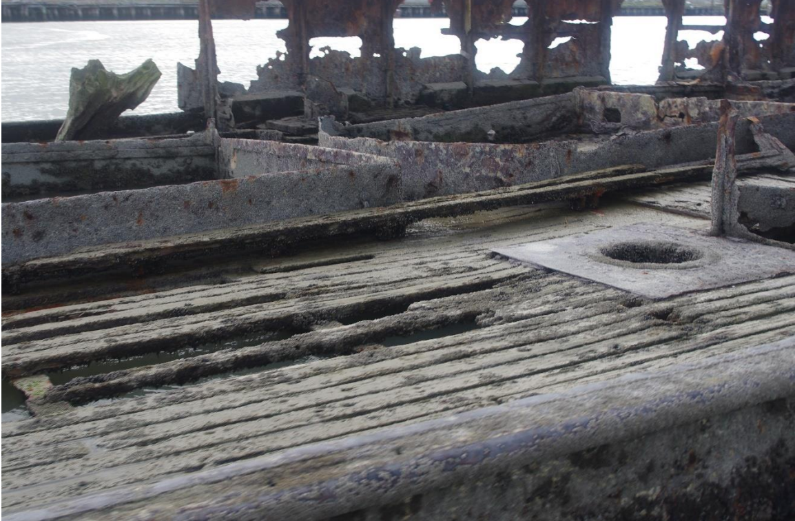
Figure 101: ss Te Anau hulk, insitu decking near bow (15.07.2021)
