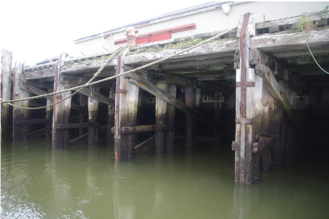
Figure 78: No.3 wharf arrangement of fenders (15.07.2021)
