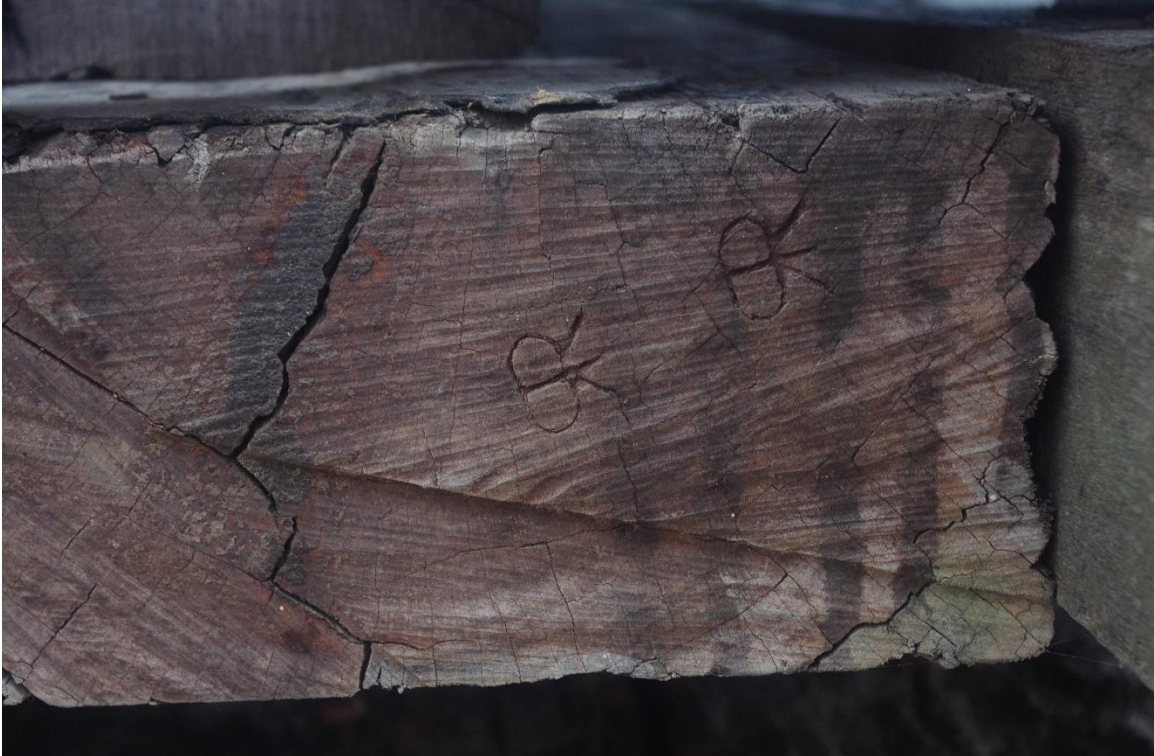
Figure 61: Stock pile, deck joist. Cutters mark? (15.07.2021)
