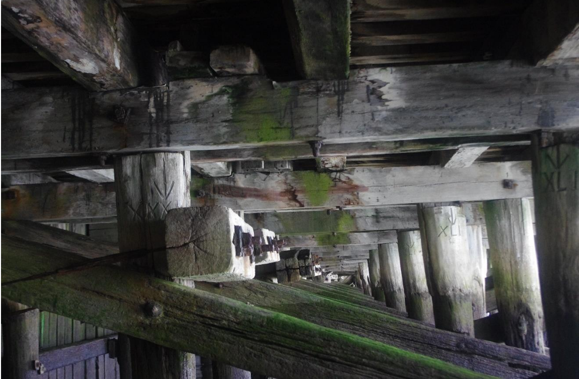
Figure 87: No.3 wharf, pile depth indicators (15.07.2021)
