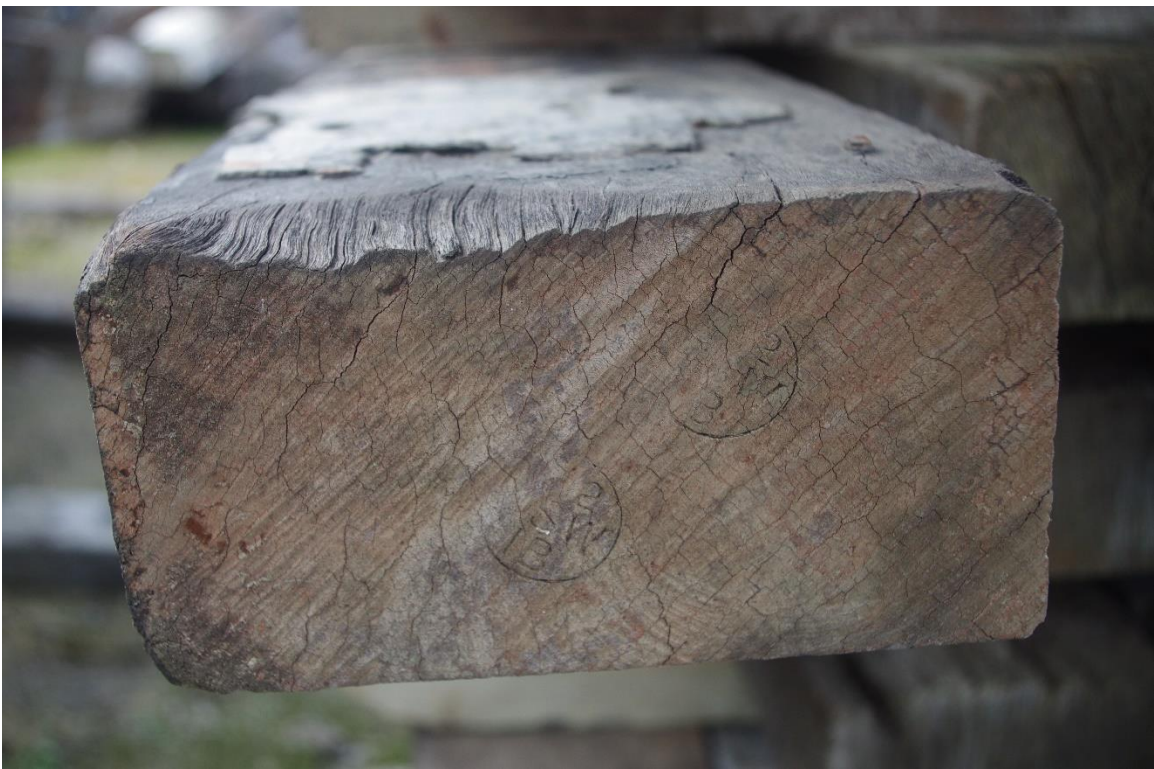
Figure 58: Stock pile, deck joist. NSW Government mark IB (Iron Bark), inspector 12 (15.07.2021)
