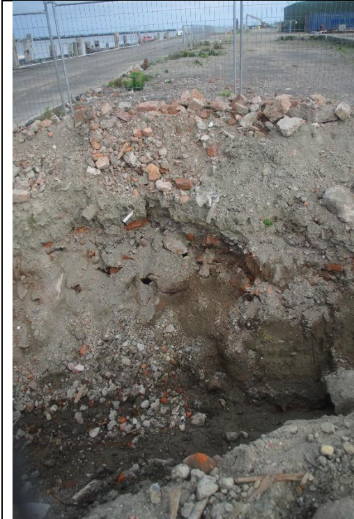
Figure 67: Interface between fill and natural soil below red shed foundations (15.07.2021)
