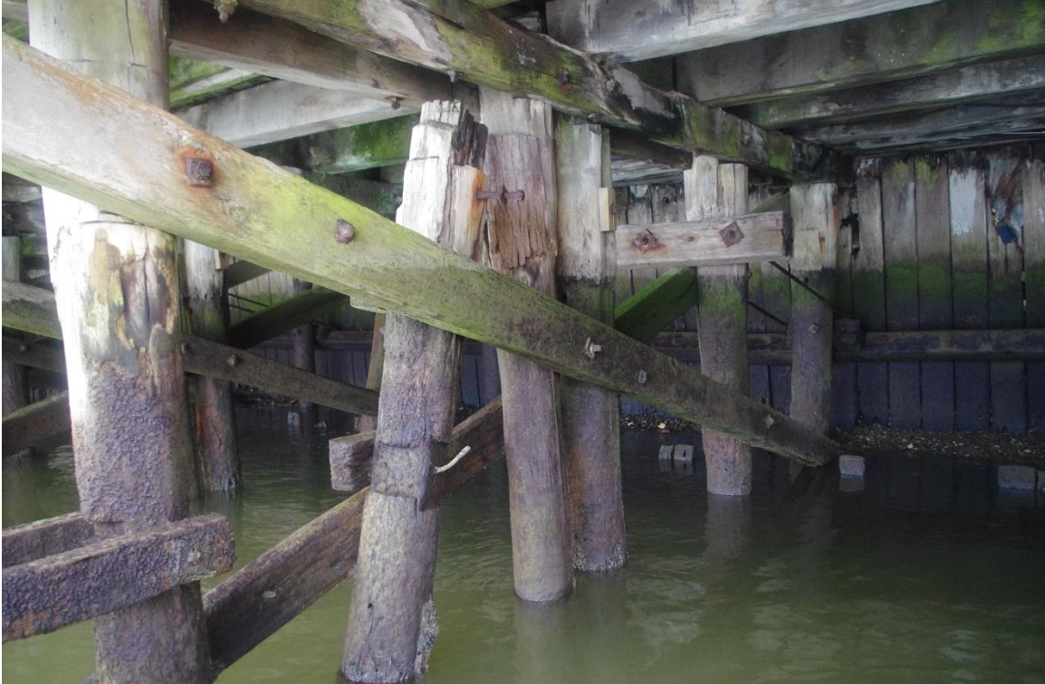
Figure 75 No.3 wharf typical arrangement of bent (15.07.2021)
