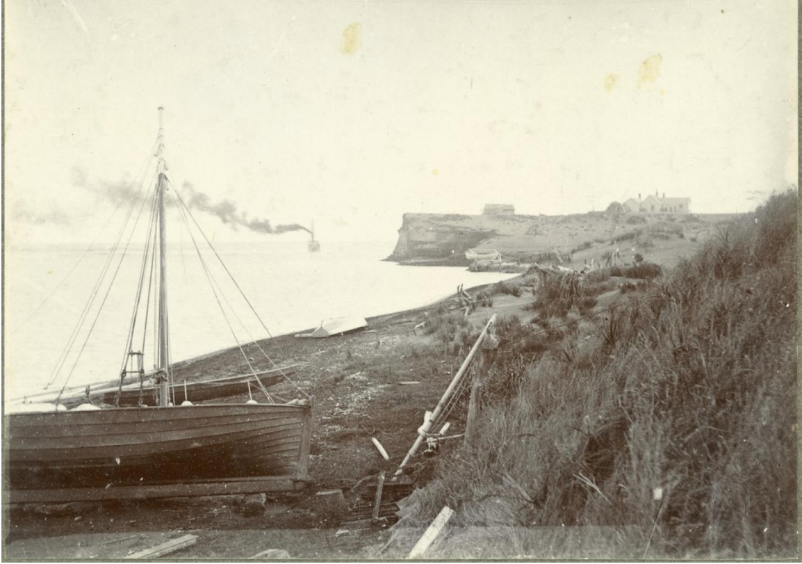
Figure 14: Early photo of Castlecliff prior to construction of wharf (Harding & Denton Collection, Wanganui District Library NZC 2.1.141)
