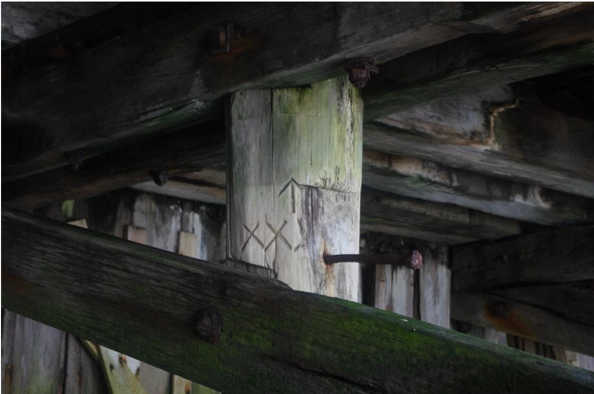
Figure 74: No.3 wharf incised roman numerals to indicate depth of driven piles (15.07.2021)
