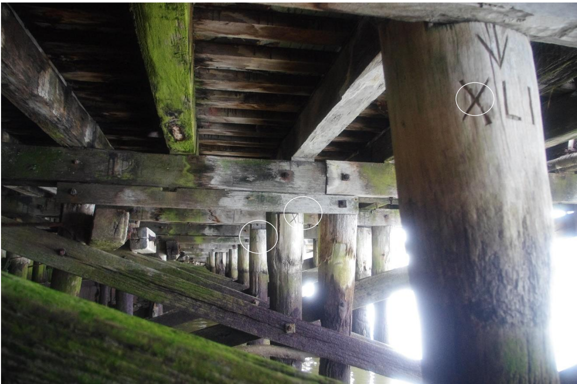
Figure 86: No.3 wharf, pile depth indicators (15.07.2021)
